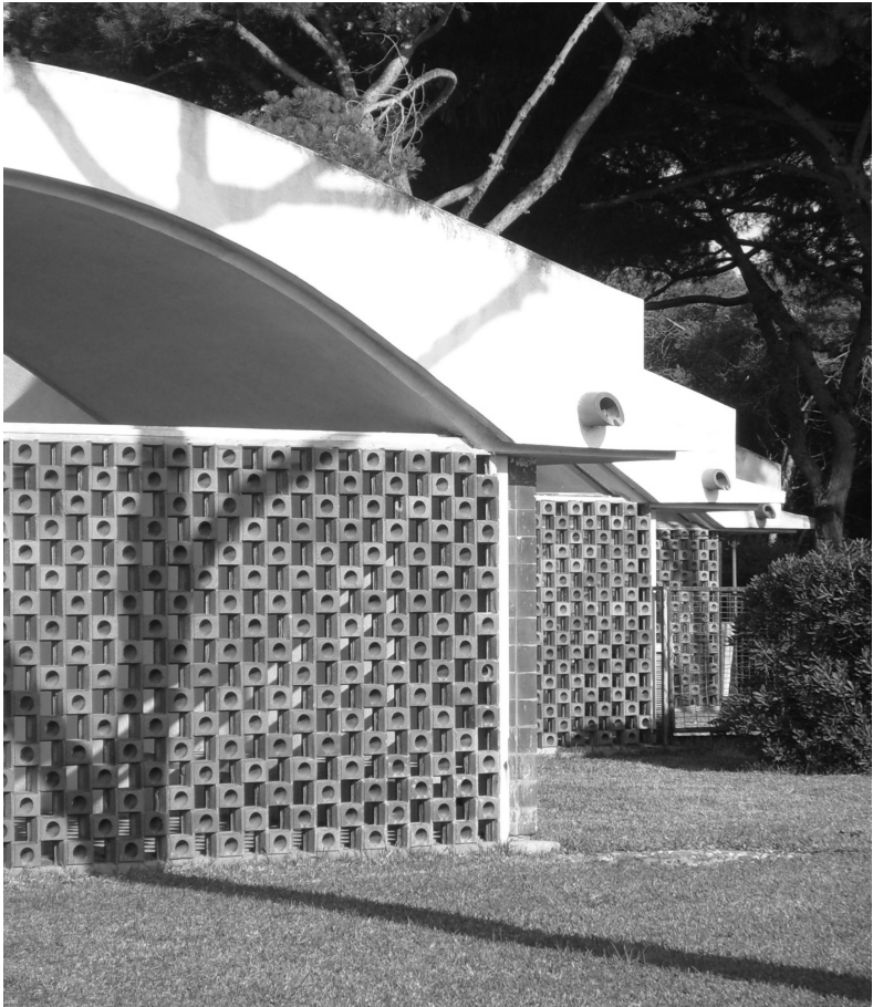
Fachada, detalle. Facade, detail.
